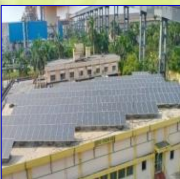
Roof of Control Room
