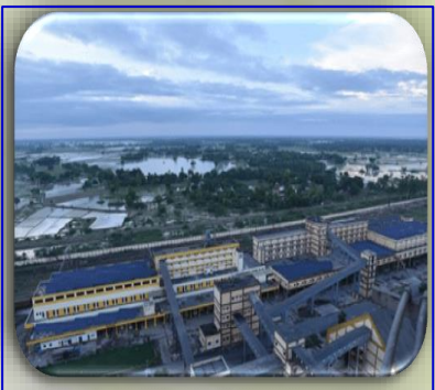
Bagging Top Floor
