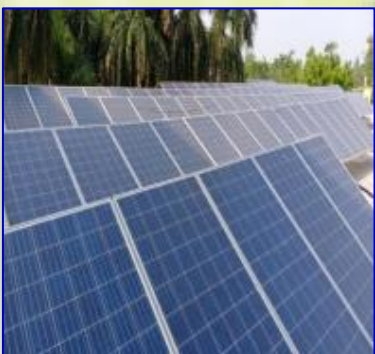
Roof of Central Canteen
